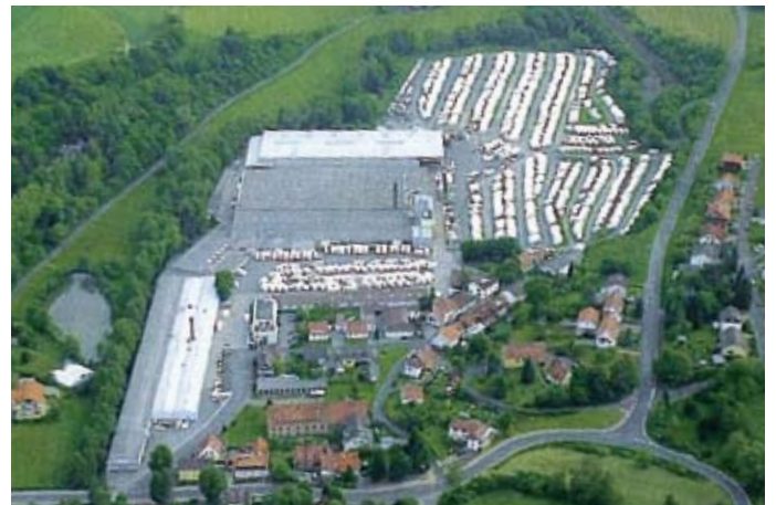
Bird's eye view of the Mottgers plant.
